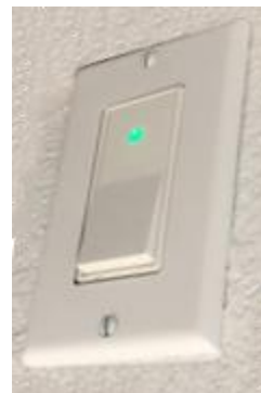
LED rocker switch installed in wall plate
